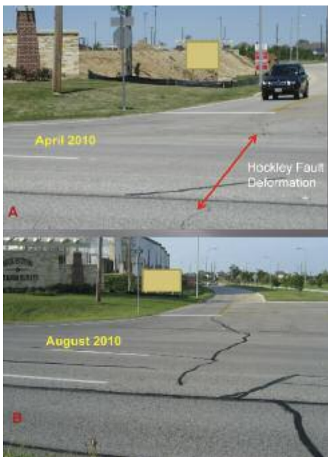
Figure 2. Recent pictures of Hockley Fault at Hwy. 290 Frontage and Fairfield Falls Way roads: A) taken in April 2010; B) taken in August 2010. Note the development of the tiny cracks in picture A into significant ones in picture B.
