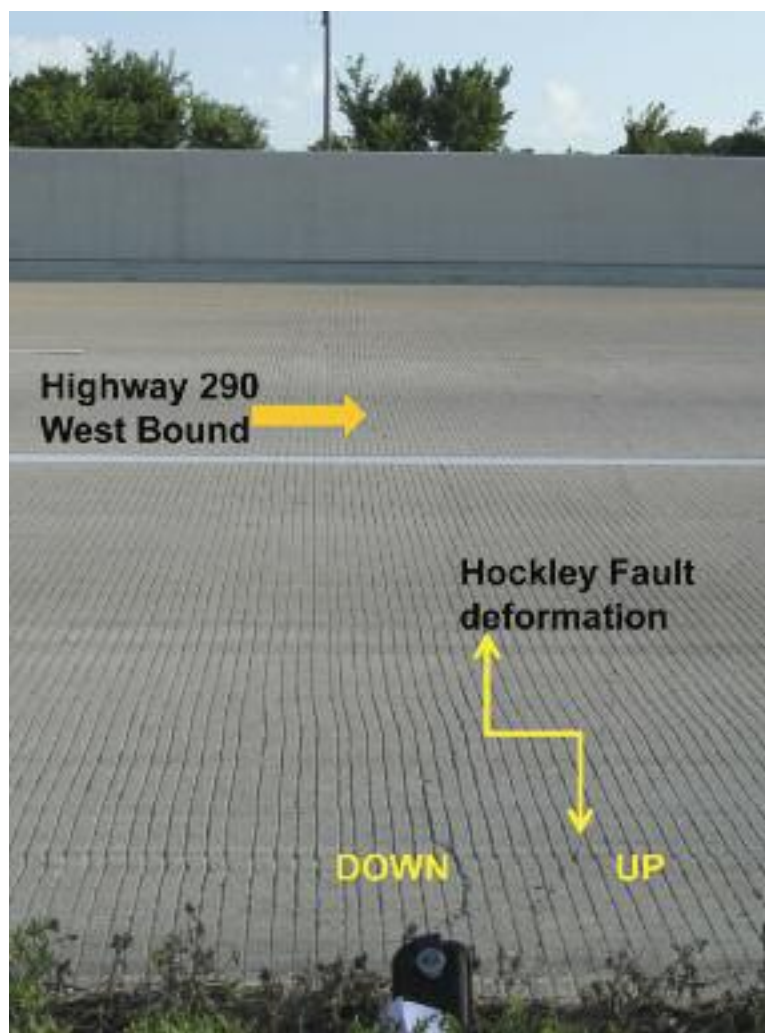
Figure 4. A recent picture (August 2010) showing revived cracks (main Hockley Fault) on the west bound of Highway 290. The fault deforms the newly built highway 290 and the feeder roads. The picture was taken facing south.
