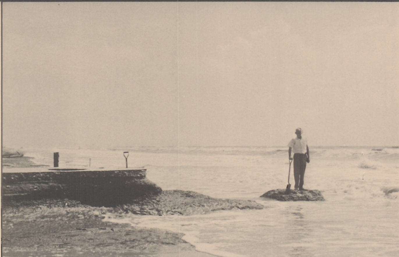
EROSION OF ASPHALT ROAD BY TRANSGRESSIVE GULF OF MEXICO
