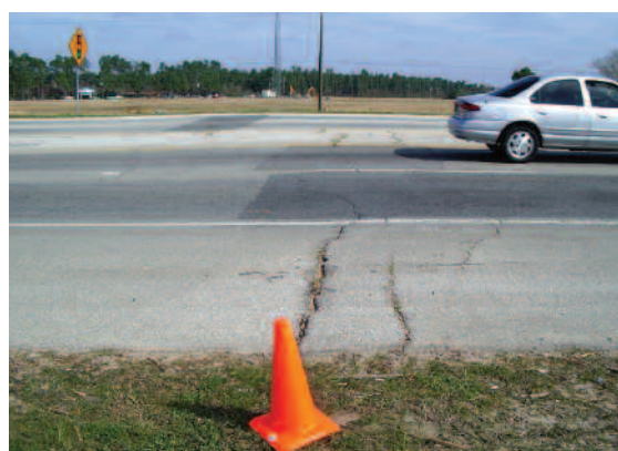
Fig. 3. View looking east of the trace of the Willow Creek fault as it crosses Highway 249. The fault is marked by the pavement cracks and asphalt patches.
