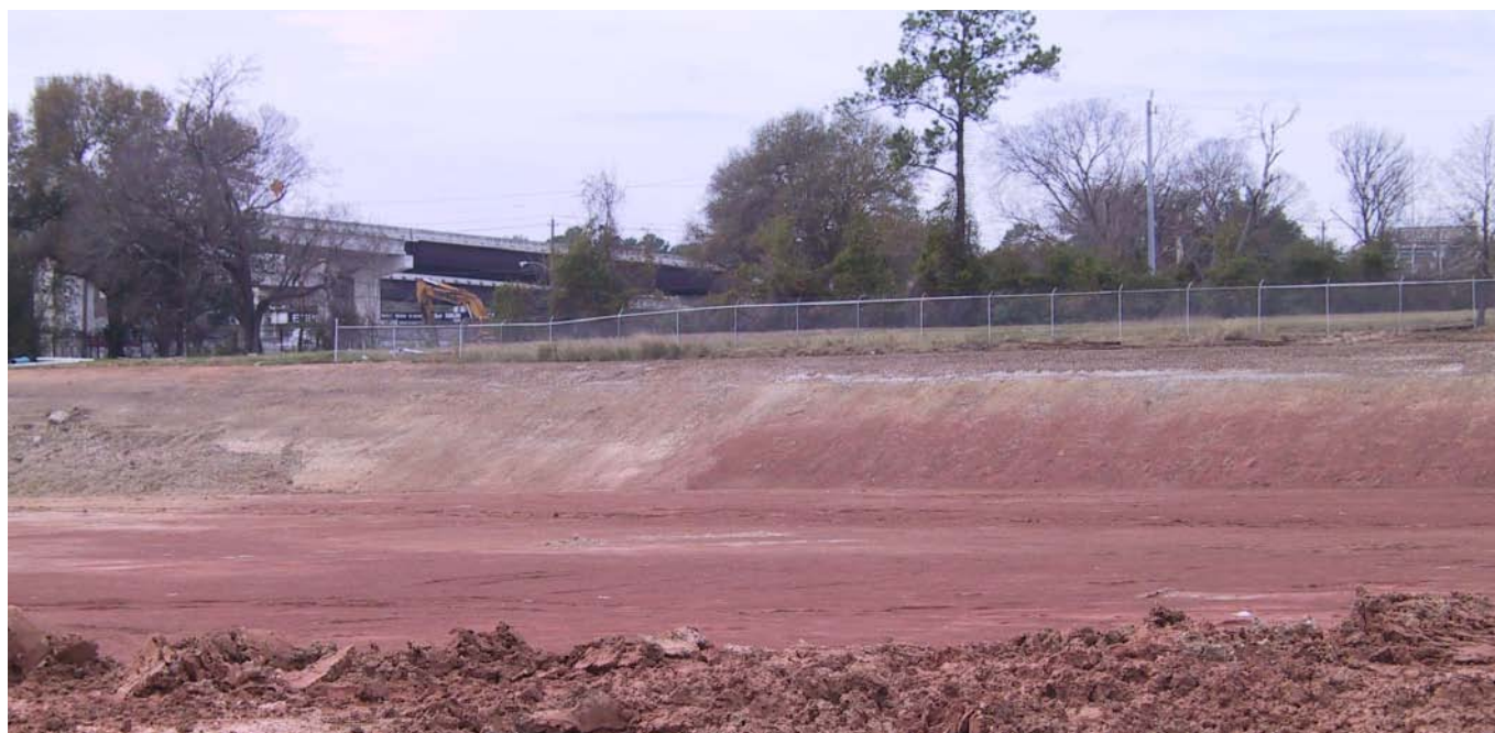
The west side of the detention pit showing the discoloration defining the fault blocks.
