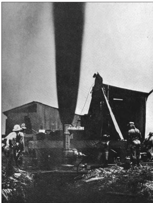
Valve completely over the well, only nine days after the blowout.
