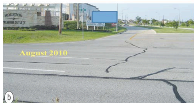
Figure 14. Recent pictures of Hockley fault at Highway 290 Frontage and Fairfield Falls Way roads: (a) taken in April 2010 and (b) taken in August 2010. Note the development of the tiny cracks in (a) into significant cracks in (b).
