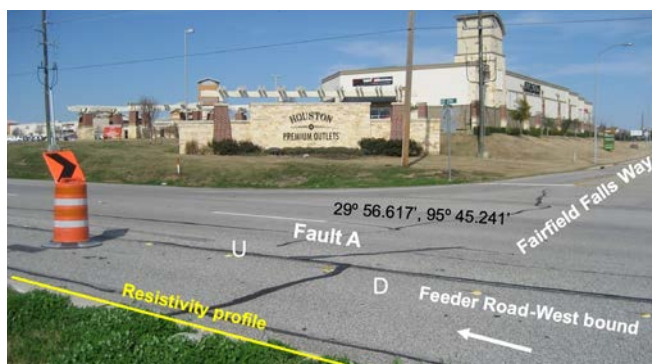
Figure 12. Photo showing the location of Hockley fault (Location A) at the intersection of westbound feeder road and Fairfield Falls, where the Premium Outlets shopping mall is located. The fault is evidenced by the cracks across the feeder road. These cracks are regularly fixed and are sometimes covered with asphalt patches. Look for deformation to the foundation of the store visible in the background. The fault crosses the West and the East-bound lanes of Highway 290. The yellow line indicates the location of the resistivity profile.
