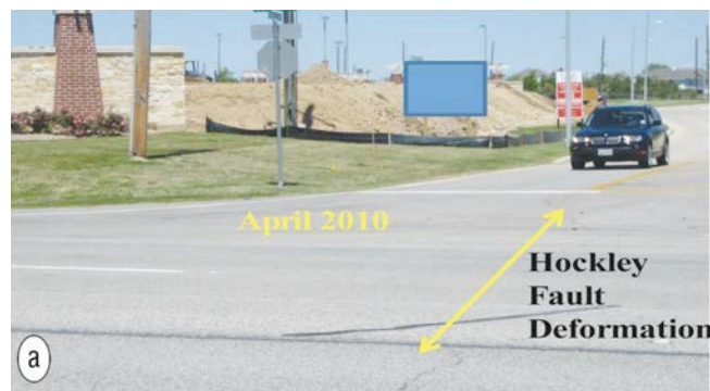
Figure 12. Photo showing the location of Hockley fault (Location A) at the intersection of westbound feeder road and Fairfield Falls, where the Premium Outlets shopping mall is located. The fault is evidenced by the cracks across the feeder road. These cracks are regularly fixed and are sometimes covered with asphalt patches. Look for deformation to the foundation of the store visible in the background. The fault crosses the West and the East-bound lanes of Highway 290. The yellow line indicates the location of the resistivity profile.
