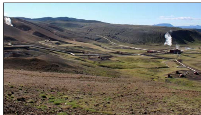
Figure 2. Krafla 60 MW geothermal powerplant located in northern Iceland showing insulated well heads and above ground pipelines on the north flank of an active volcano.
