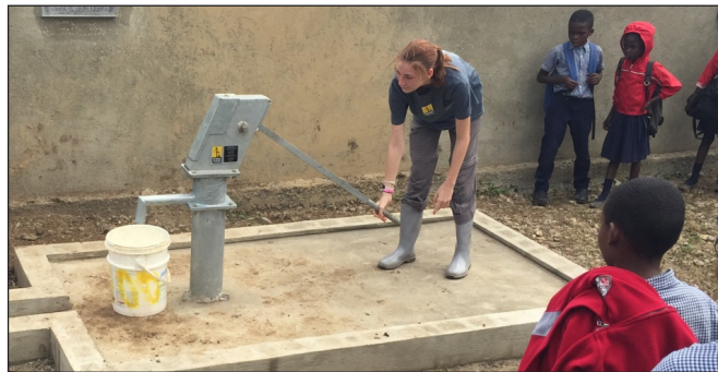
Katie Meinen testing the newly installed pump
